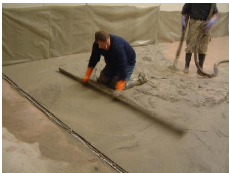
Striking off with straightedge/aluminum lath
