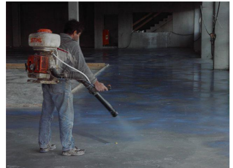
Curing with KOROSEAL
