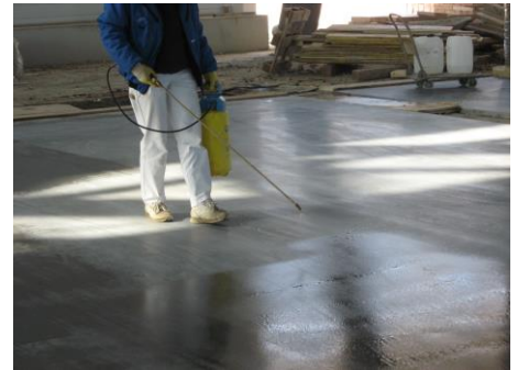
Curing with KOROTEX
